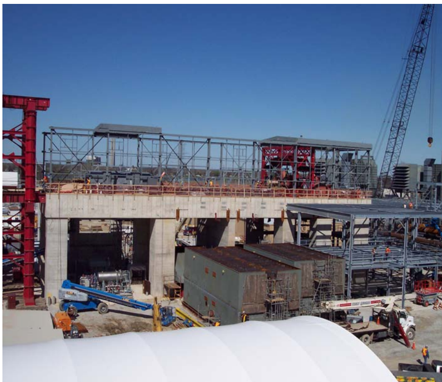
The condenser being installed
