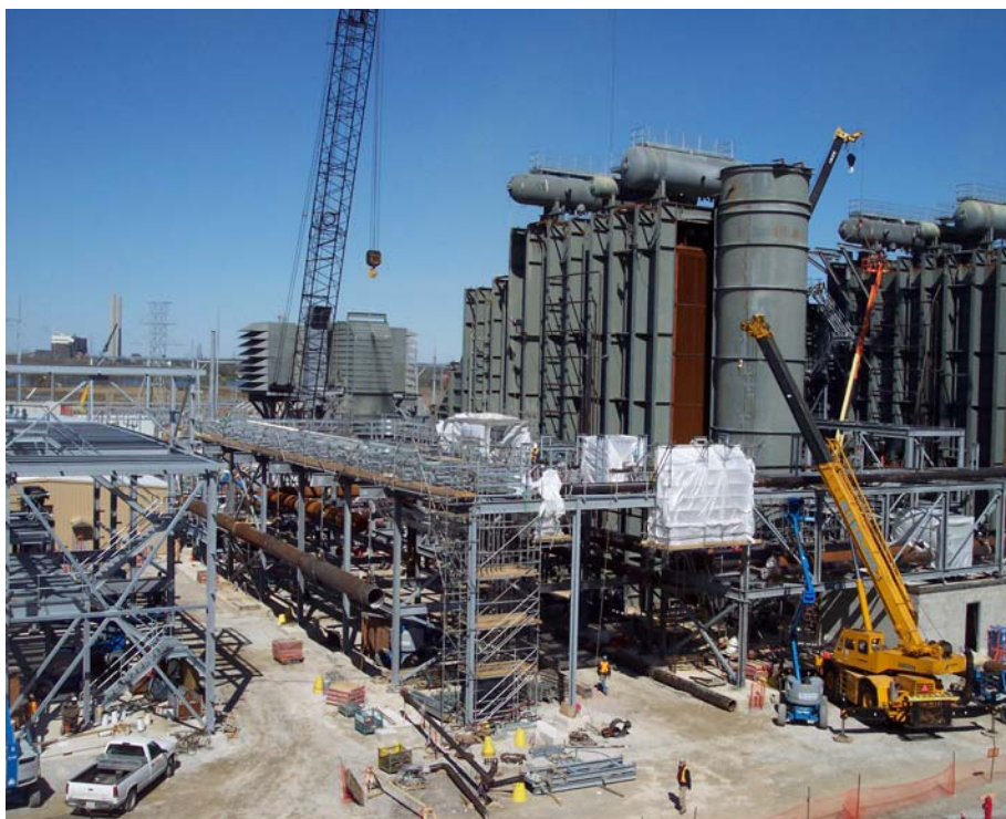
The steam header being put in place
