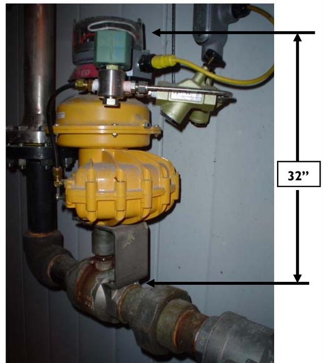
**Figure 2.0 2" Bracket & Coupling Technology**
