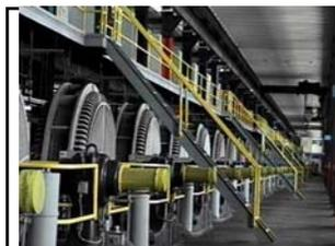
A/C generators which produced power at 25 cycles
